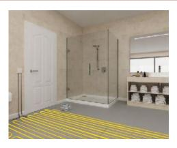
Prepare floor plan of the area to be heated and identify suitable location of the fused spur and thermostat position - mark the layout of the underfloor heating mat on the floor plan.
