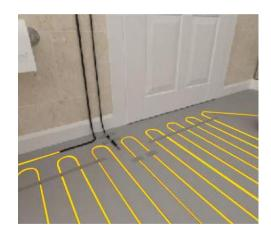
Now start installing the floor heating mat from the thermostat position. Roll out and secure the mat to the floor. The heating mat has a sticky mesh, simply press this down onto the floor and it will hold in place. If you need to turn the mat 90 degrees upside down you can use the double sided adhesive strips to hold the mat in place. A small amount of additional cloth tape is provided to ensure the mat is flat to the floor in places where it is uneven.
